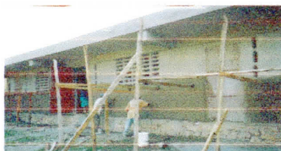
Surfacing the walls
